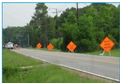
Signage notifies residents of underground construction activities.
